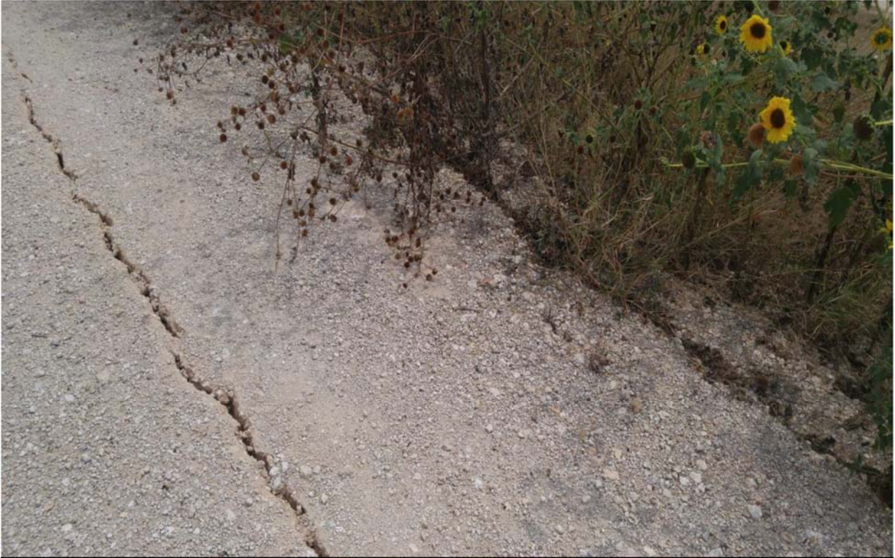
Photo 3 - Looking South - New Surface Tension Crack East of Pins 8 and 9
