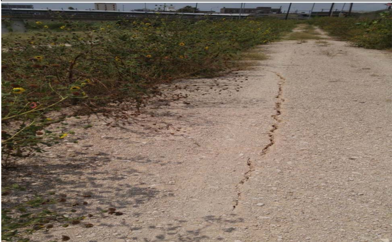
Photo 2 - Looking North – New Surface Tension Crack East of Pins 8 through 11
